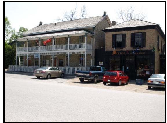
Figure 3: An example of well maintained buildings in the district
