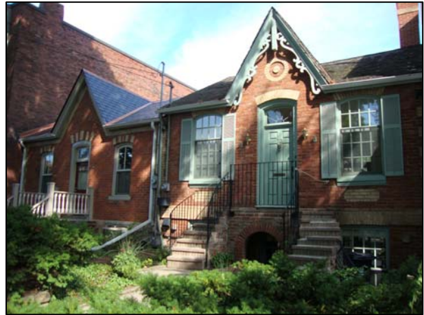
Figure 3: Well maintained buildings.
