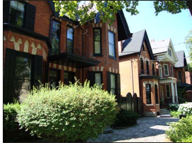
Figure 3: Examples of well maintained buildings
