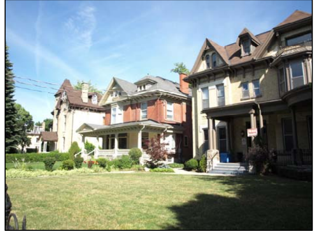
Figure 3: Example of well maintained houses.
