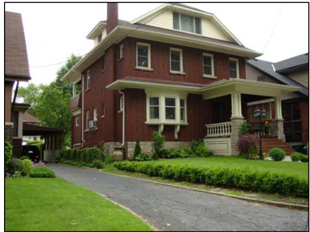
Figure 3: An example of the well maintained streetscape including historic buildings as well as private and public plantings.
