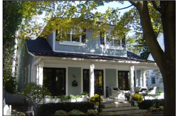
Figure 3: An example of a building in view with high scores in façade quality and conservation work
