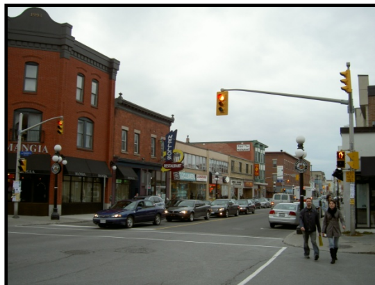
Figure 3: An example of well maintained buildings
