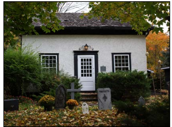
Figure 3: An example of a building in view with high scores in conserved elements and facade quality
