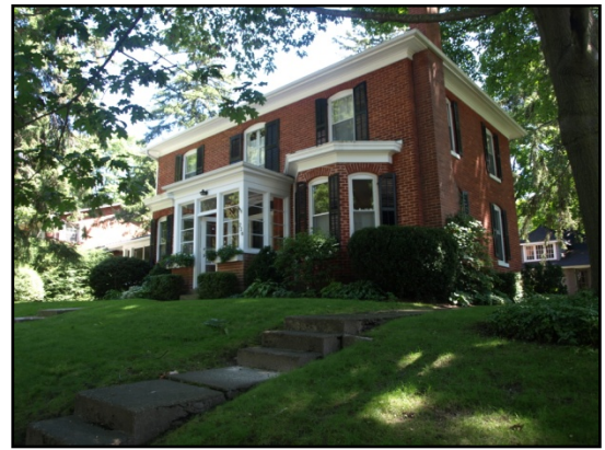
Figure 3: An example of a building in view with high scores in facade quality and conservation work
