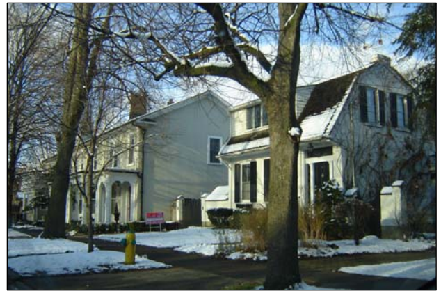
Figure 3: An example of well maintained buildings
