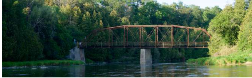
Figure 31. Steel truss bridge on Township Road 60
