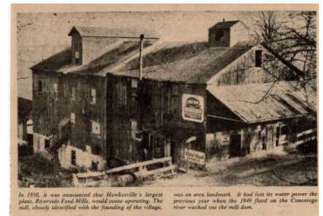
Figure 20. An image of the Hawkesville feed mill before it was demolished. This image was submitted by a participant to the interview method (I281).
