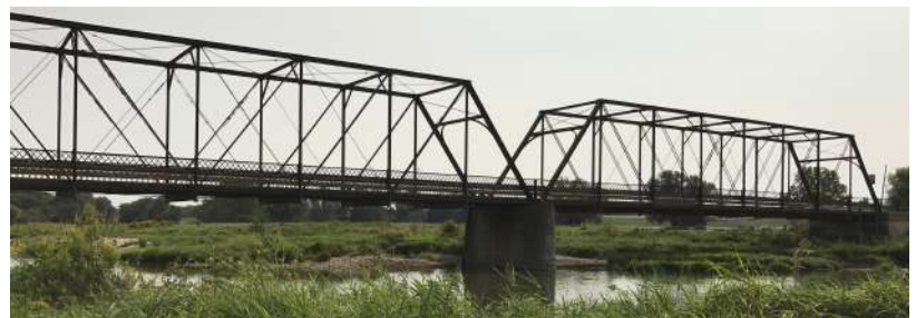
Figure 30. Image of Glasgow Street bridge, Conestogo.
