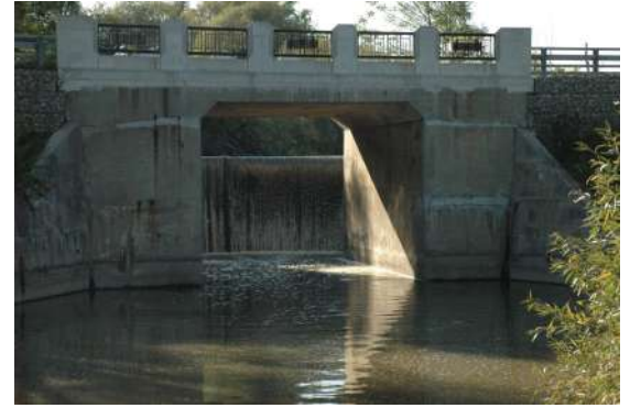
Figure 37. Image of the dam located under Floradale Road.
