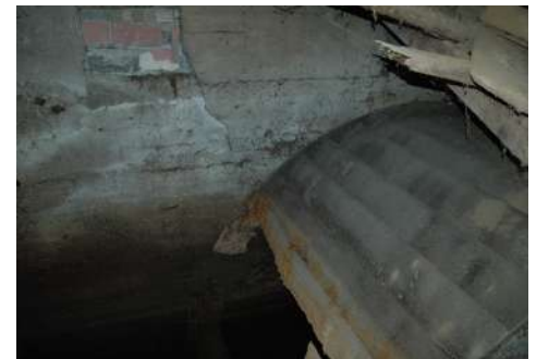
Figure 38. Remnants of the large overshot wheel constructed by Daniel Bowman.
