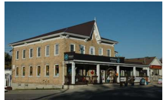
Figure 58. This building once served as the St. Clements Hotel and Tavern.
