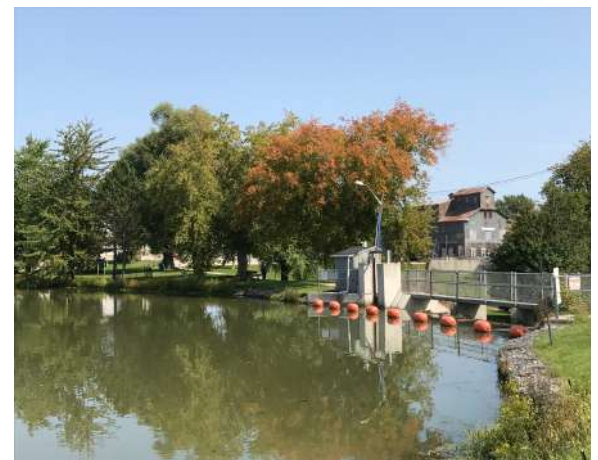
Figure 73. The Wellesley dam with the previous site of the Doering Grist Mill in the background.
