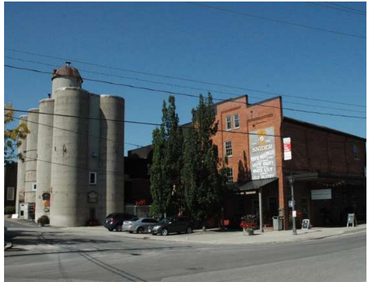
Figure 67. A prominent feature of the St. Jacobs streetscape is the mill located at the north end.
