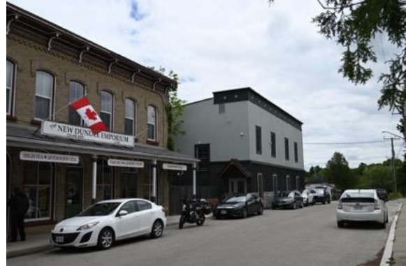
Figure 40. View of the Emporium and streetscape, facing south on Front Street.
