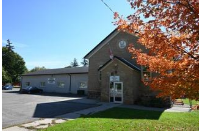
Figure 12. New Hamburg School Section 6, located in New Hamburg and currently being used as the New Hamburg co-operative preschool.
