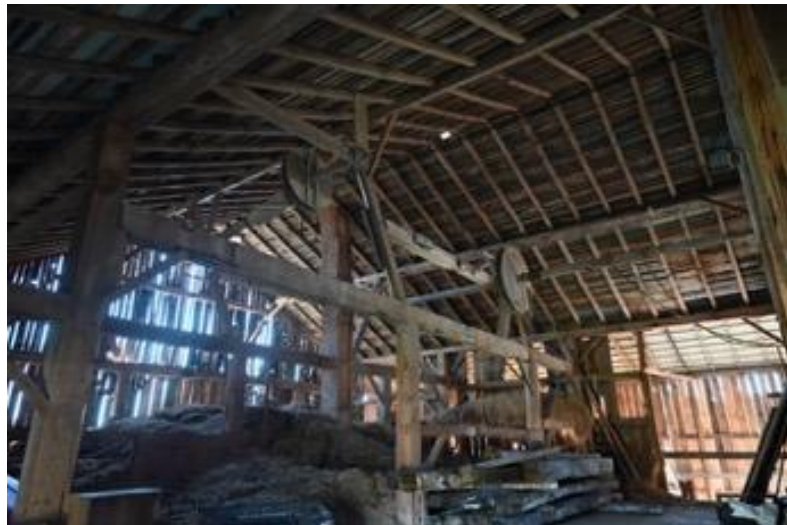
Figure 11. View inside a barn immediately west of Pinehill Cemetery. Note the single beam spanning the width of the barn.
