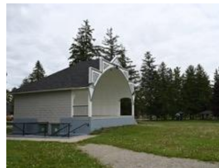
Figure 39. The New Dundee Bandshell located in the New Dundee Community Park.
