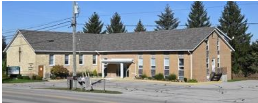
Figure 10. View of Rosebank Church.
