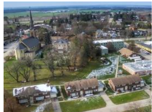
Figure 70. An aerial photograph of the Canadian Independent College located adjacent to St. Agatha Church and Rectory (sourced from https://cicwaterloo.ca/ ).
