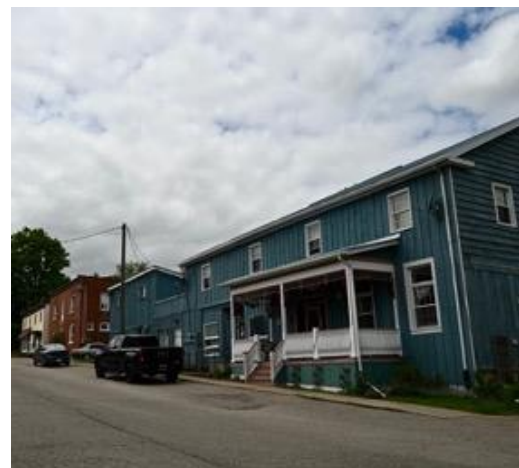
Figure 36. View of the downtown streetscape of New Dundee.
