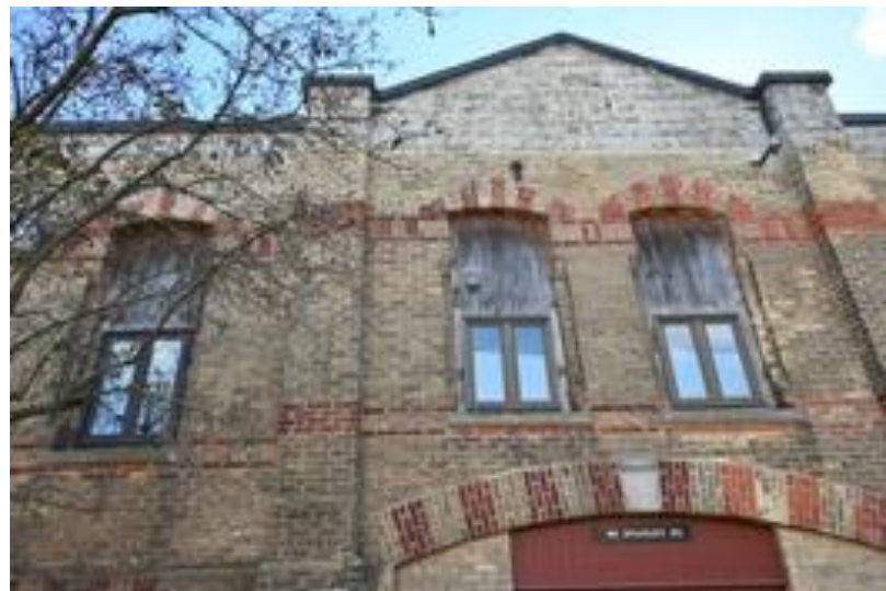
Figure 87. Former Watson Foundry.
