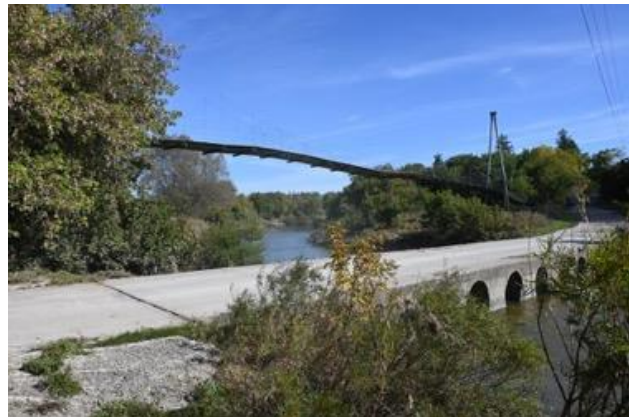
Figure 42. Two bridges spanning the Nith River, north of Christner Road.
