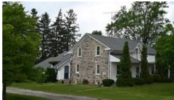
Figure 48. The Shantz House at 2632 Erb's Road.
