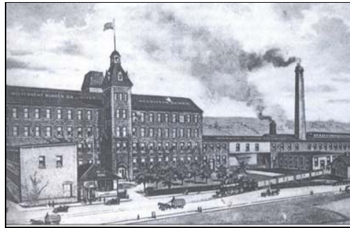
Before the great fire of the 1960s destroyed the larger part of the mill
