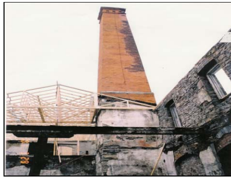
A new roof and repairs to the chimney
