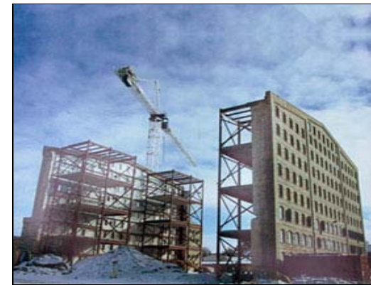
Process of demolition- construction in the case of the Seagram Lofts
