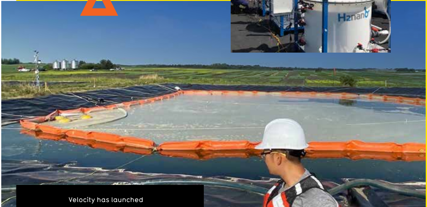
© H2NANO'S TECHNOLOGY PROVIDES A REUSABLE, CATALYZED REACTION TO CREATE TREATMENT COMPOUNDS FROM CONTAMINATED WATER. PHOTO COURTESY OF H2NANO.
