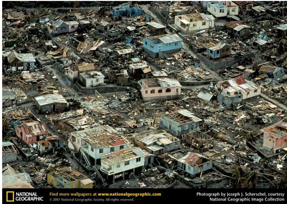
Picture 6.1: Damage Caused by Hurricane David (1979)
