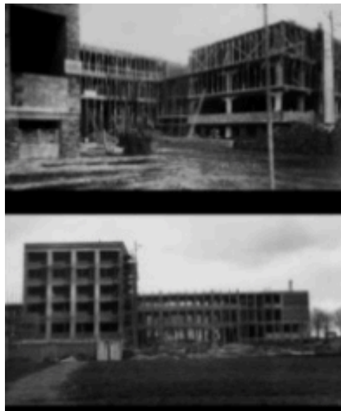
Figure 1: The Dessau Bauhaus, under construction. +/- 1925
