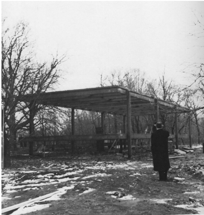
Figure 2: Lutz Mies, contemplating a steel frame
