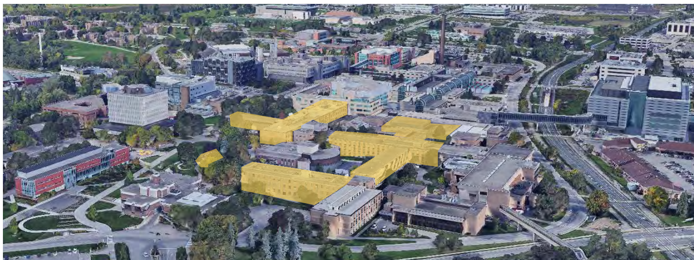
Figure 12. Aerial image of campus from southeast, with early buildings annotated in yellow, 2025 (Google Earth; annotation by Brook McIlroy)
