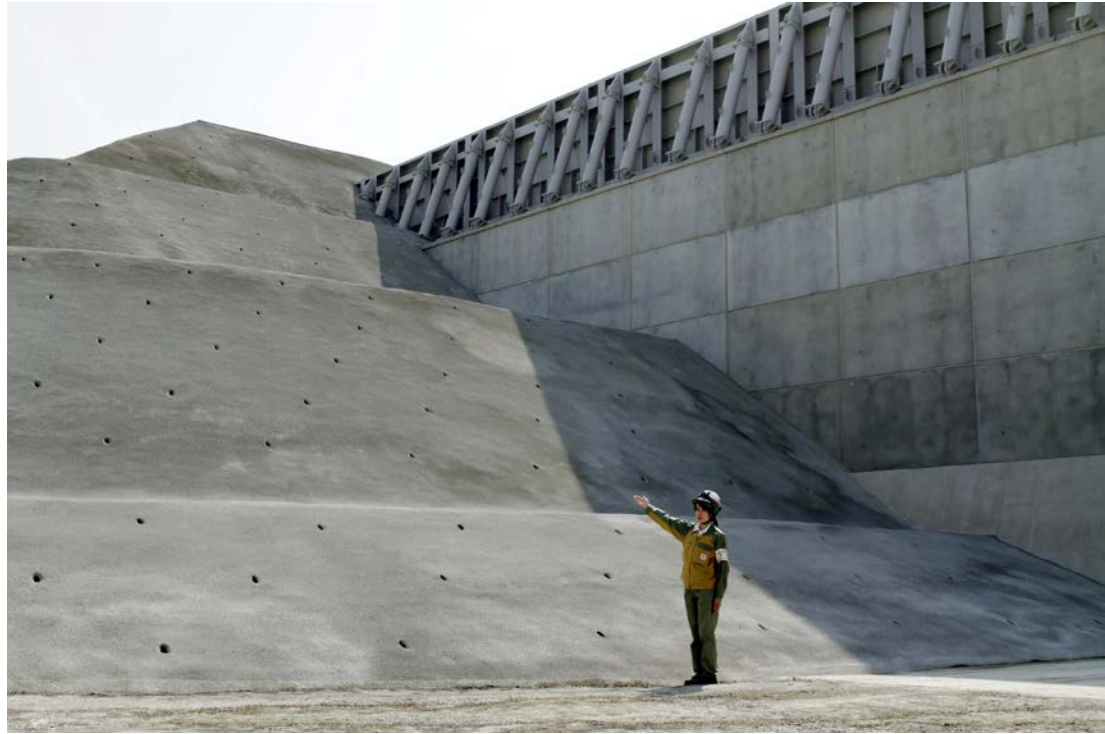
Tsunami Sea Wall. Hamaoka, Japan. www.japantimes.co.jp/news/2016/03/31/national/sea-wall-guard-tsunami-completed-hamaoka-nuclear-plant/
