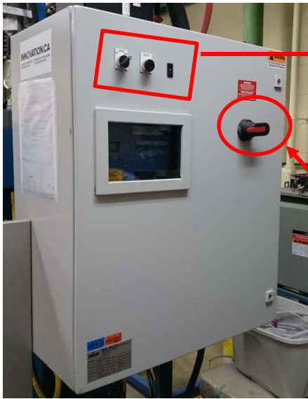
Switch lever • Showing "OFF" position • Turn clockwise (90 degrees downward) to switch "ON"
