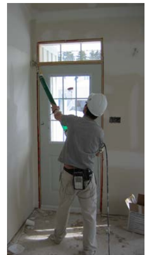
Finishing drywall using pneumatic drywall finishing system
