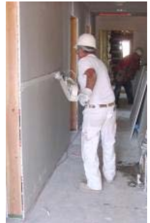
Finishing drywall using traditional mudbox
