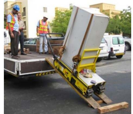
Transporting supplies to worksite using the all terrain dolly
