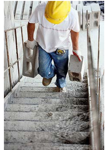
Manually transporting materials up stairs
