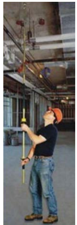
Anchor Jack (Picture courtesy of Tebmar Products Inc.)
