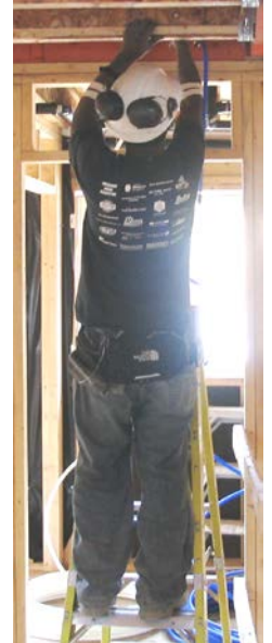
Traditional method of manually crimping pipes.
