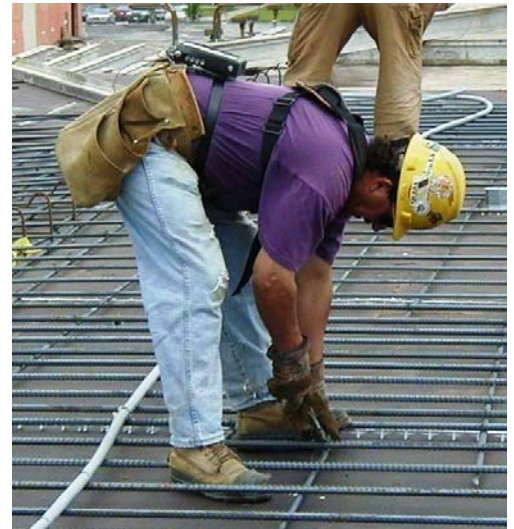
Tying rebar by hand
