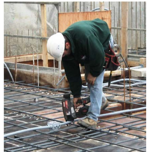
Tying conduit to rebar using a mechanical tying tool.
