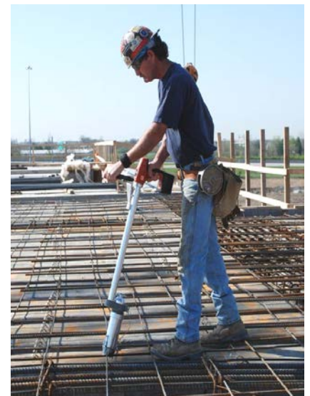
Rebar-tying tool with coiled spring wire handle
