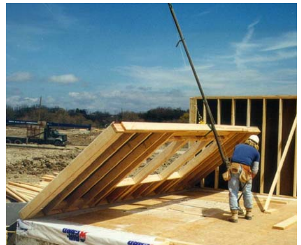
Lifting wall with a hydraulic lifter.
