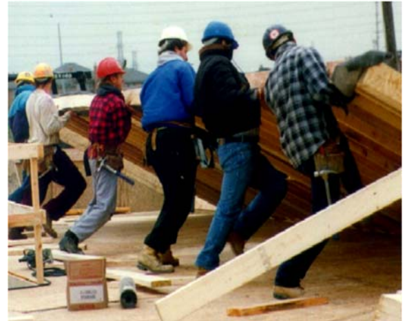
Manual wall lifting
