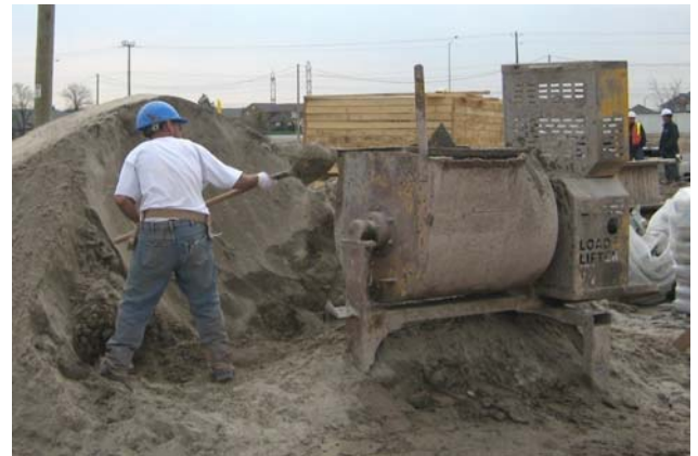
Traditional method of transporting grouting using buckets.
