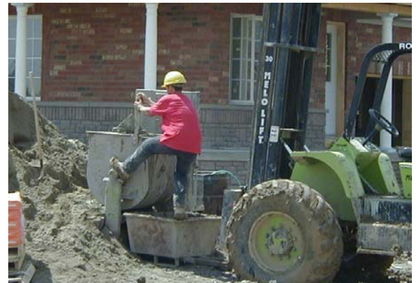
Traditional method of manually dumping the product from the mixer drum into tub.
