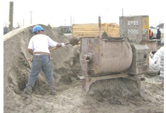
Traditional method of shoveling sand into a mixer.
