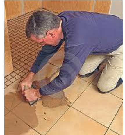
Kneeling on floor while grouting tile
