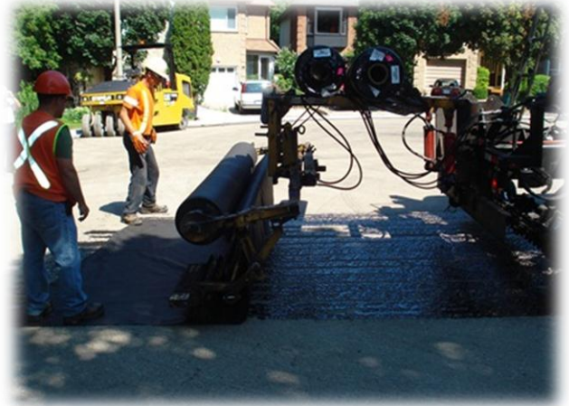
SAMI – Placing GeMat on Emulsion for SAMI application
