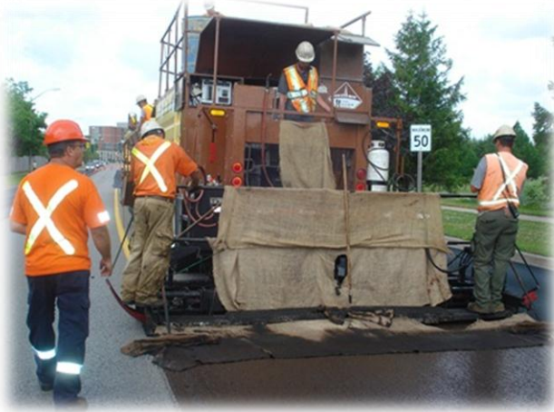
Microsurfacing – Placing Emulsion Mix
