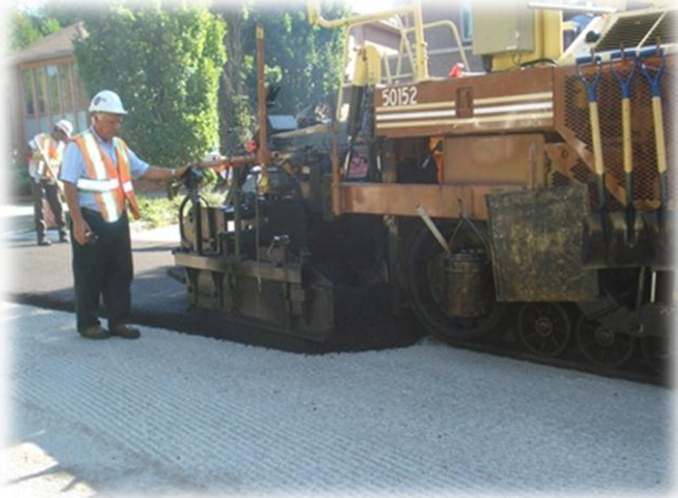
Paving – Placing 50mm Asphalt
