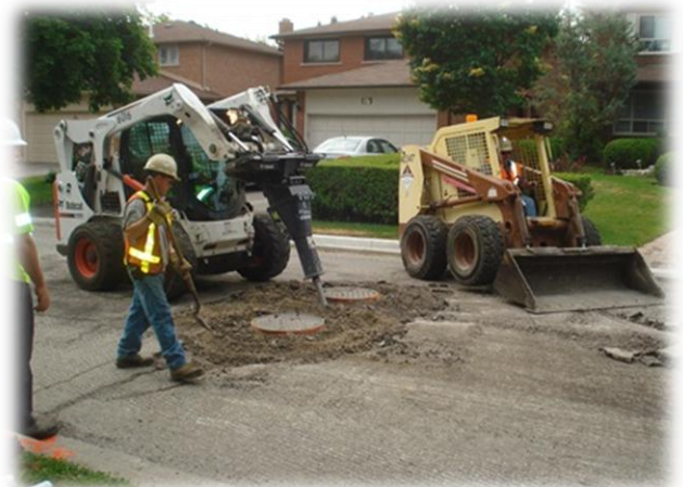
Shave and Pave – Preparation for Lowering Manholes
