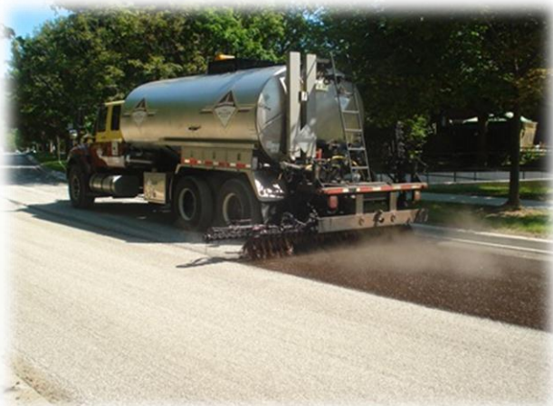
SAMI – Placing emulsion on GeMat for SAMI application
