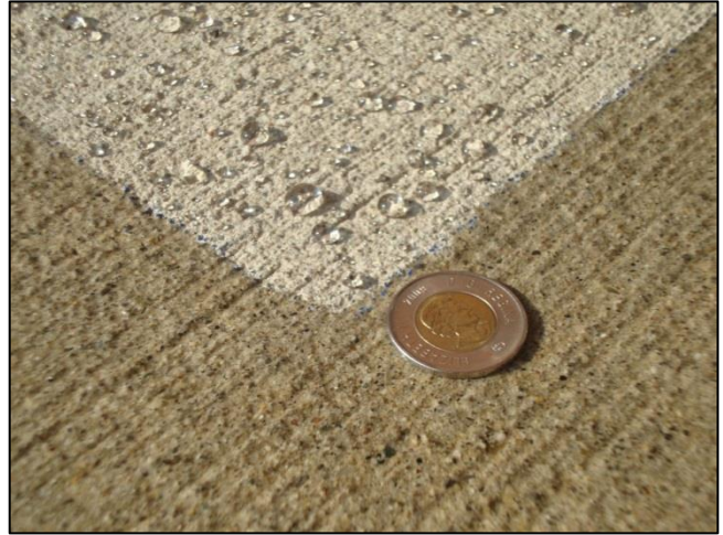
Nano lotus leaf effect on concrete pavement – broom finishing – 0% slope
