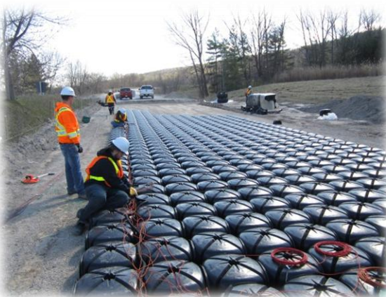
Concrete embedment strain gauge sensor installation
