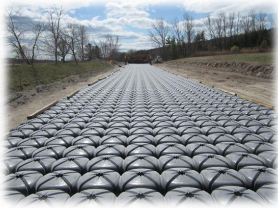
Cupolux all set up prior to paving
