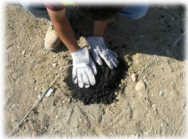
Asphalt Strain Gauge Installation
