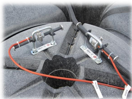
Strain gauges mounted on Cupolex prior to paving
