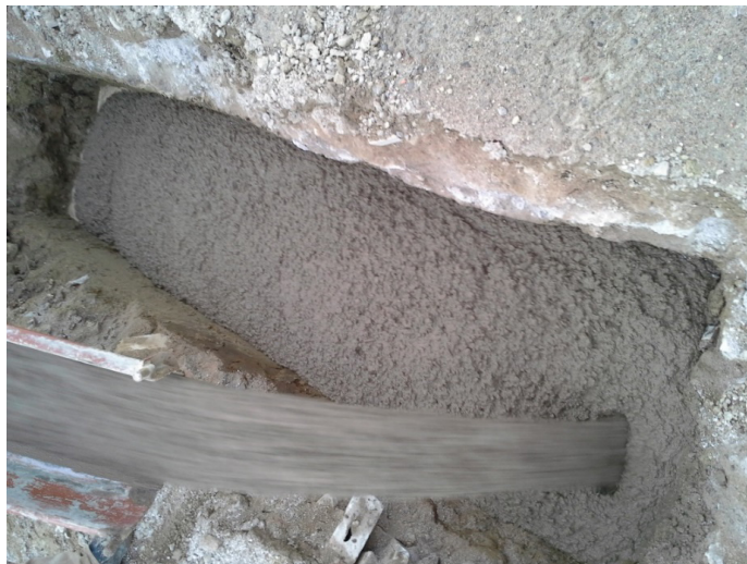
Placement of u-fill during field trials
