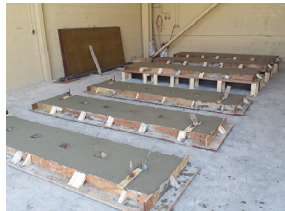
Specimens after casting (precast with stud pockets)
