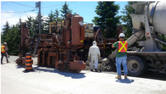
Concrete overlay being placed at Spragues Road, Region of Waterloo
