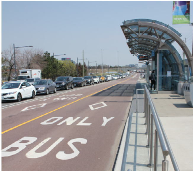
Highway 7 BRT-Lane, York Region, Ontario, May 2015
