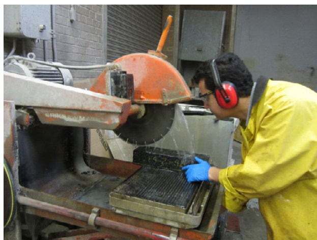
Saw cutting of HMA Beams and Preparation
