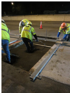
Precise technique for placing levelling material
