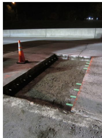
Repair area ready for placement of Super-Slab
