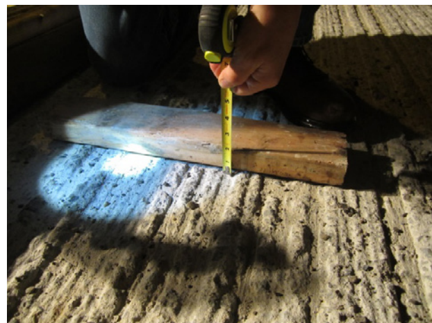
Surface texture of milled surface
