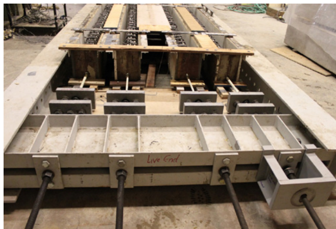
Formwork placed inside the prestressing bed
