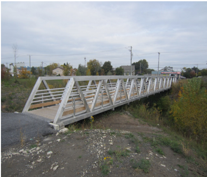
Daigneault Creek Bridge
