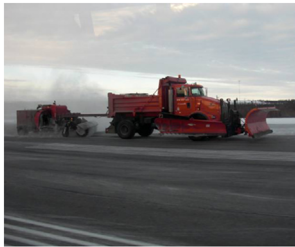
Runway winter maintenance activities - brooming operations
