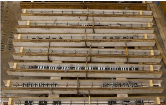
Beam specimens with different simulated spalling conditions, ready for concrete casting
