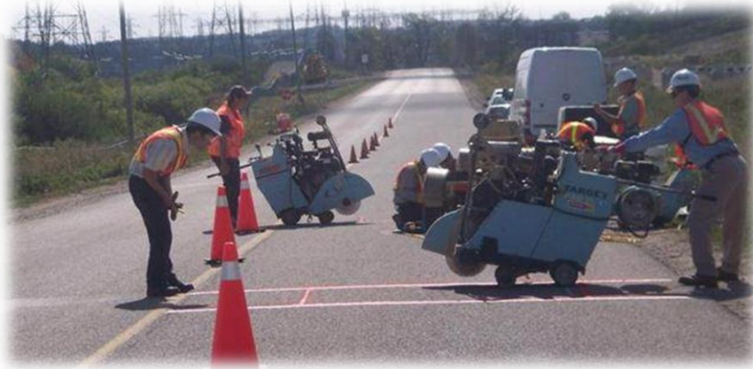
WIM Installation at Landfill, September 2007
