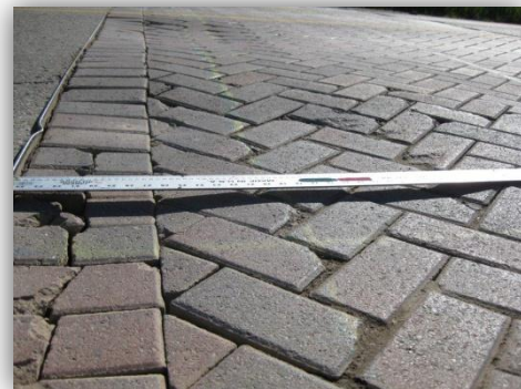
Monitoring Performance of Crosswalk Field Sites
