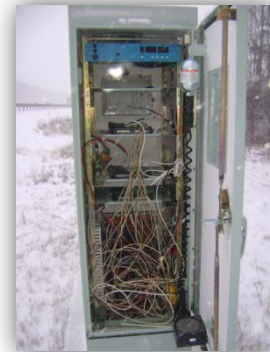
Collecting Data from Instrumented Perpetual Pavement on Highway 401
