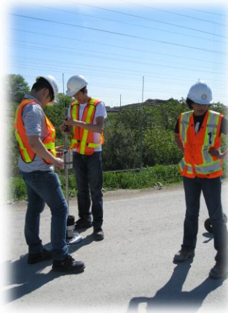
Portable Falling Weight Deflectometer (FWD) Testing
