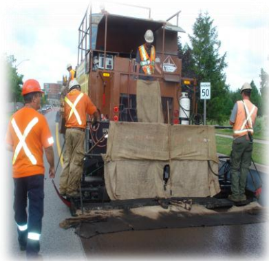
Placing Emulsion Mix in the Town of Markham
