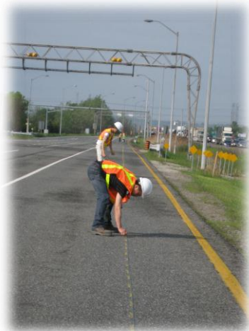
Marking pavement for SurPro testing
