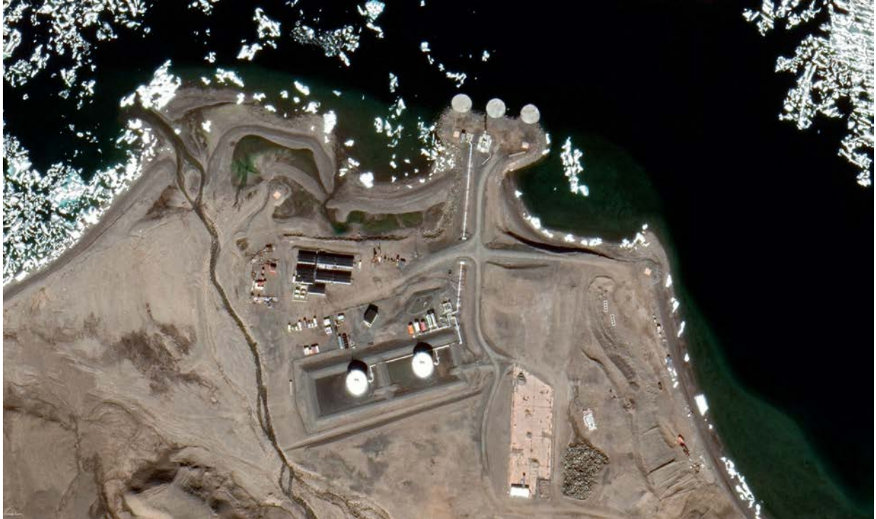
Fig. 4: Nanisivik Naval Station, the much-delayed naval refueling station (in Admiralty Inlet off Lancaster Sound at the north end of Baffin Island) is nearing completion. Google Earth
