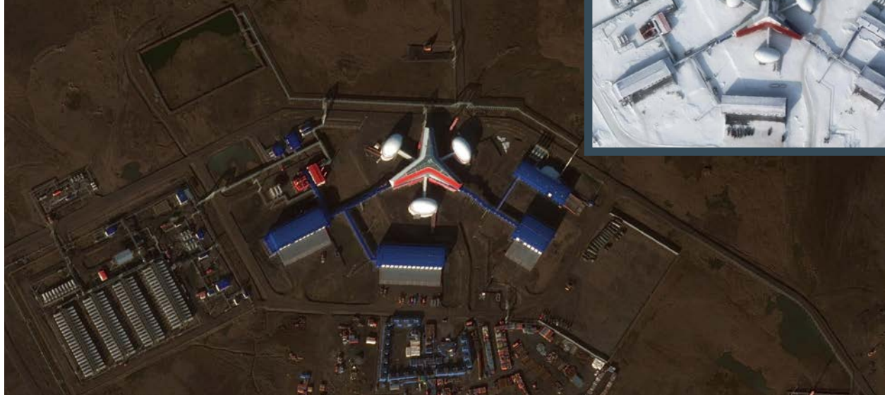
Fig. 17: Franz Josef Land's "trefoil" facility (with winter scene inset) is barracks and operational centre base for the Nagurskoye base. SecureWatch
