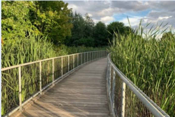
Boardwalk and viewing platform.
