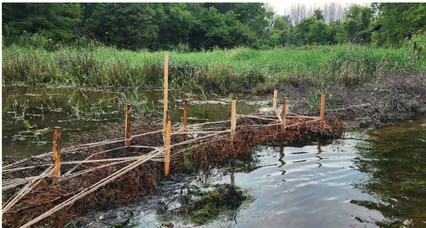
Figure 5. Stream restoration event using donated Christmas trees led by Conservation Halton on August 1, 2024. Photo by Alison Clarke.
