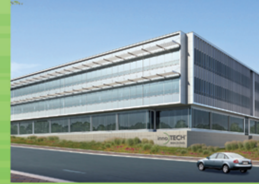
InnoTECH Building • Research + Technology Park, Waterloo
