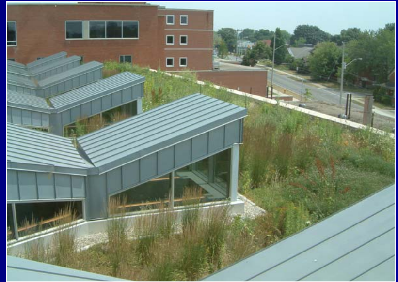
Roof Top Gardens
