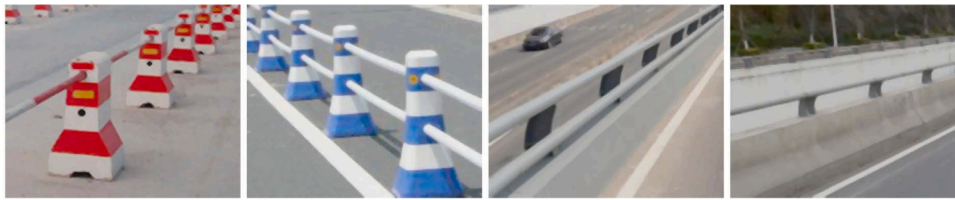
Fig. 10. Guardrails on roads. left: lane-separating; right: anti-fall guardrails (Gao et al., 2020).
