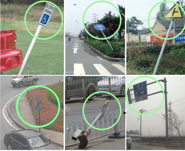
Fig. 1. Examples of traffic signs with bad placement or appearance (collected from Internet).
