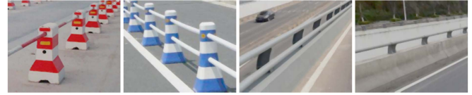
Fig. 1. Guardrails on urban roads (the lane-separating guardrails on the left and the anti-fall guardrails on the right).
