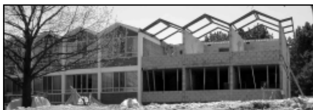
The extension to the residence building has room for 26 more students.
