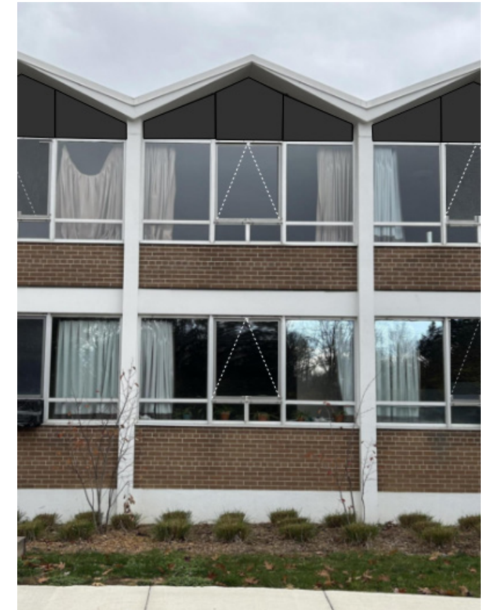
OPTION 2A: TRIPLE GLAZED WITH PEAK INFILL OPTION 2B: DOUBLE GLAZED WITH PEAK INFILL
