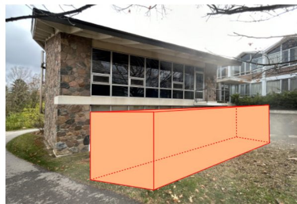
OPTION 1: AHU (Deemed non viable due to equipment size on site)
