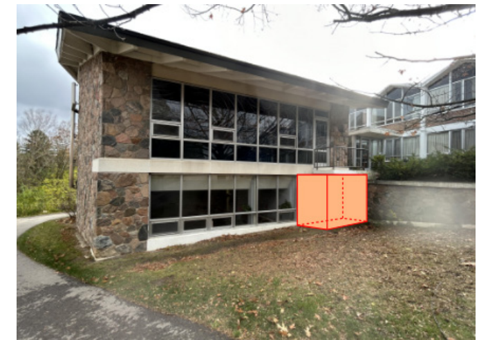
OUTDOOR CONDENSING UNIT
